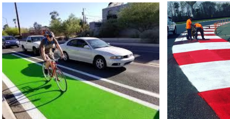
Example of textured pavement markings: crushed colored glass (Ruby Lake, 2017) and racetrack marking (Advanced Pavement Marking, 2017).
