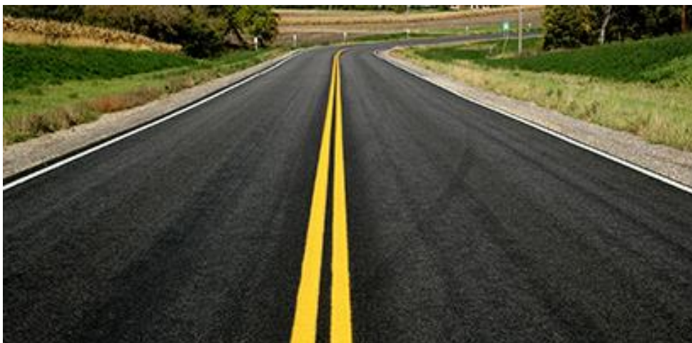
Yellow centerline and white edgeline pavement markings (3M, 2017).
