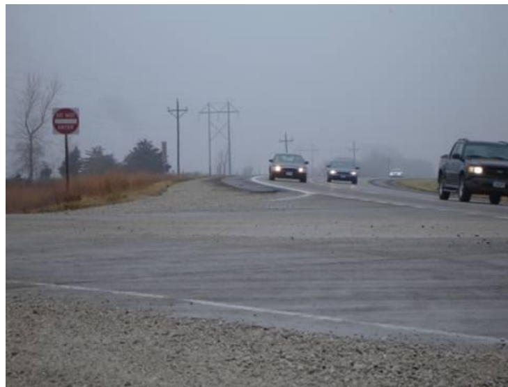
Example of superelevation on a multilane roadway (Stein & Neuman, 2007).
